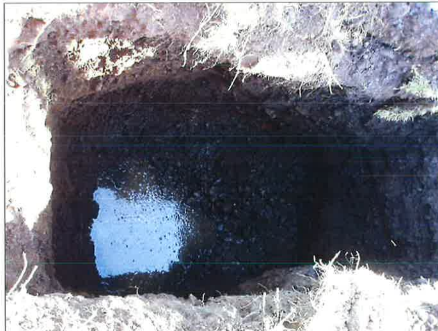
Photo 2: Groundwater Seepage in Test Pit TP3
